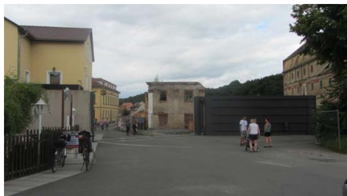
Figure 27 Floodgate, part of the floodwall Project 1
